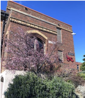
This photo was taken one week before the demolition of the front garden and entrance of the PTHS Main Building. Photo by Jan Boutillier
